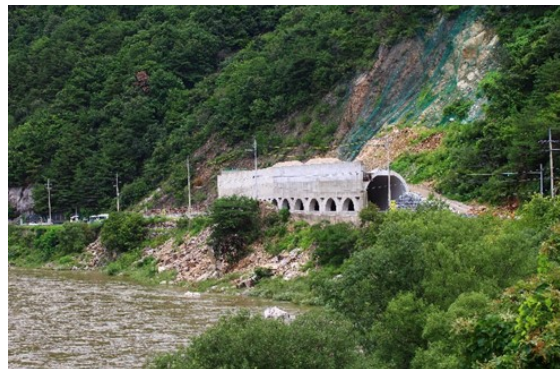
Fig. 1 Precast arch tunnel constructed in the area where rockfall occurs
