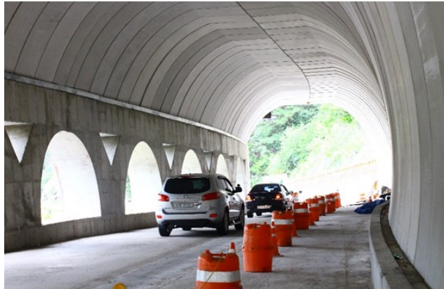
Fig. 3 Inside view of precast rockfall protection tunnel
