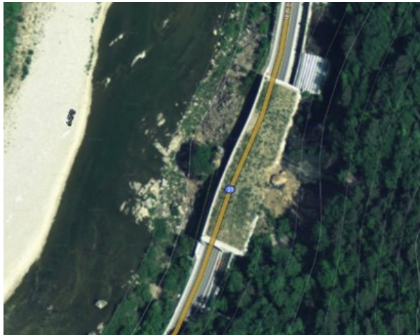
Fig. 4 Rockfall falling on the precast protection tunnel
