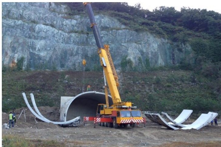
Fig. 5 Recycling of precast arch segments
