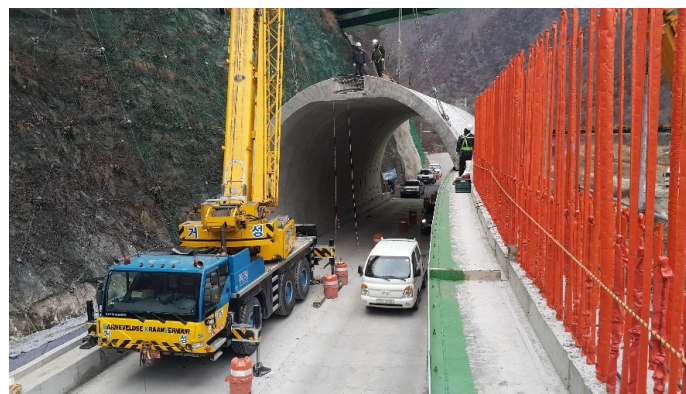
Fig. 2 Install precast arch segment while maintaining vehicle traffic
