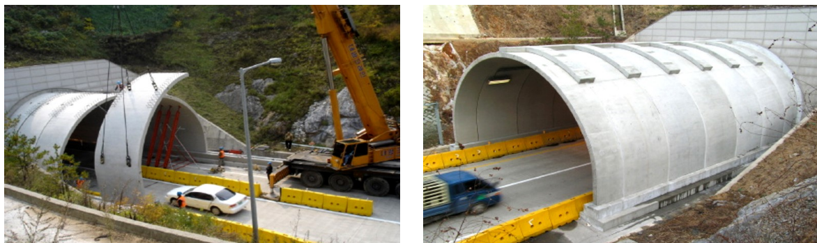
Fig. 9 Precast rockfall protection tunnel constructed at tunnel entrance
